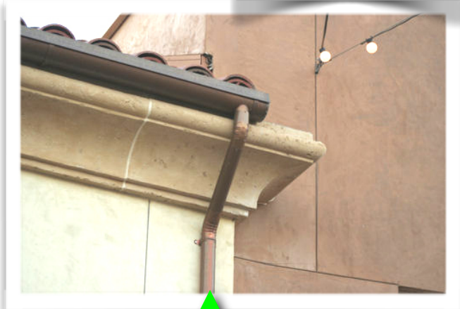
✓ DO use copper gutters and downspouts where appropriate
