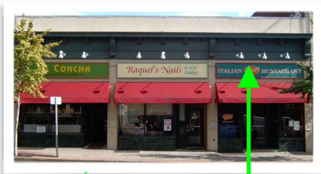
DO use parapets with cornice detailing on single-story facades to add visual
