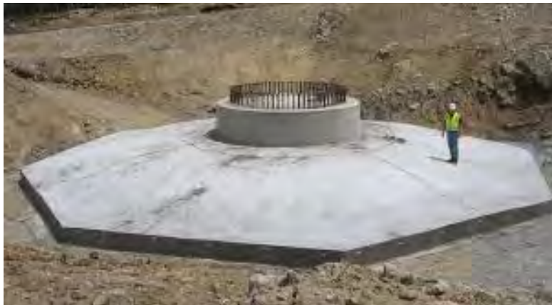
Figure 2: Shallow Foundation
